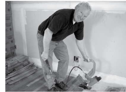
Helping the Motor City Blight Busters, Paul Johnson 100881 was our team leader helping to install the new hardwood floor.
